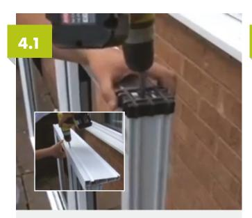
Remove any packaging from the new frame and screw the cill onto the bottom of the frame. Make sure you select a screw that will not penetrate the inner skin of the frame.
