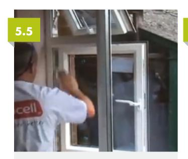
Prior to sealing the frame to the internal wall, clean the frame and glass so it is free from dirt and grit. When using cleaning agents be sure to keep the room well ventilated.
