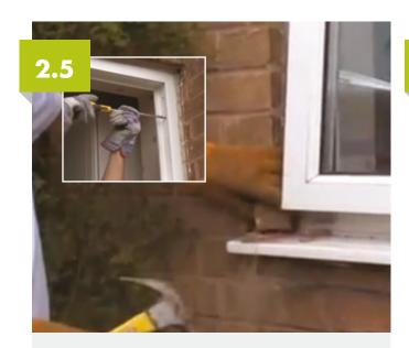
Remove and old fixings and break the external silicone seal with a blade. Also remove the external brick corners, to release the old frame.
