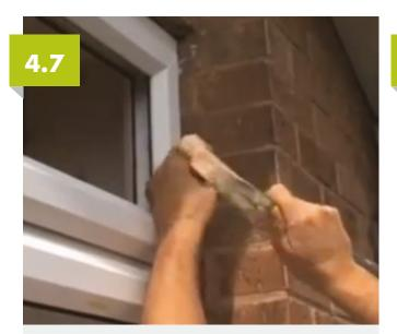
Using a chisel, break off the excess ends of the packers to create a neat finish.
