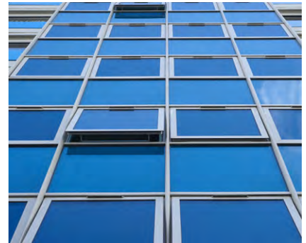
Aluminium clad curtain walling
